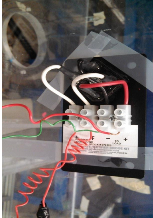
Figure 3.7 Wave Bridge with Wiring
