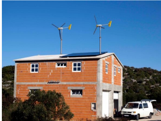
Figure 2.11 Bergey 1 KW System
