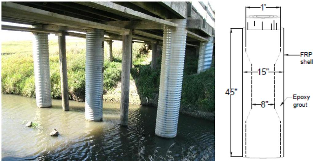
**Figure 9:** Pile Metal Jacketing, on left (Phares, 2015) and Pile FRP Wrap with Epoxy Grout, on right (White et al., 2007)
