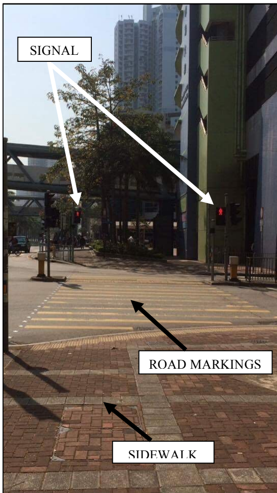
Figure 20: Safe Intersection with Signals and Road Markings in Tin Shui Wai
