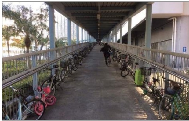
Figure 25: Bikes Chained to Fence Outside of Tin Shui Wai Station
