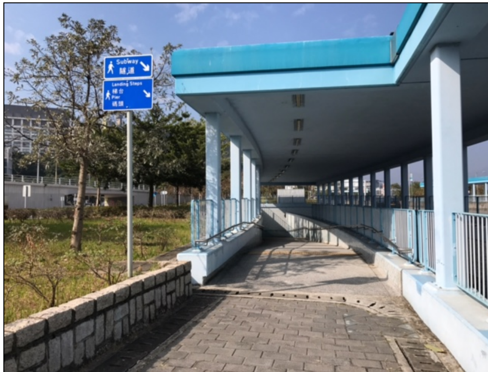
Figure 17: Subway Entrance along Bike Route to Science Park
