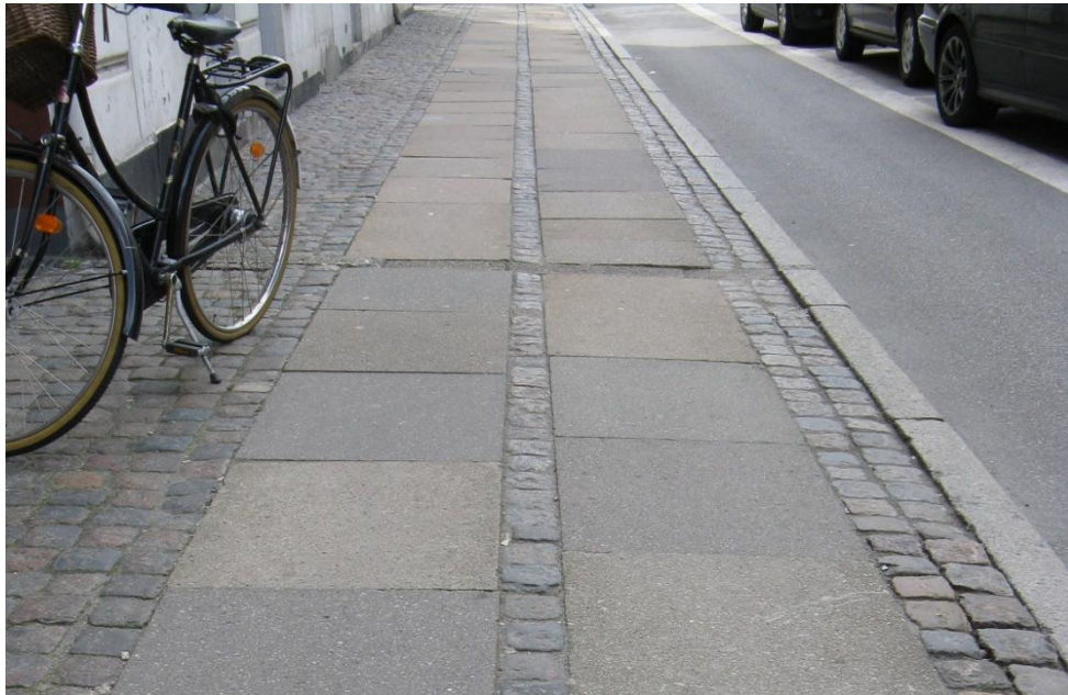
Figure 10: Sidewalk with tactile cobblestone path in Copenhagen
