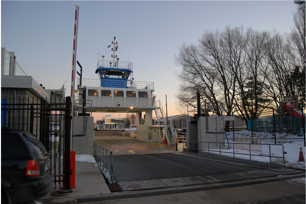
Figure 55: Many ferries use non-fixed adjustable loading ramps.
