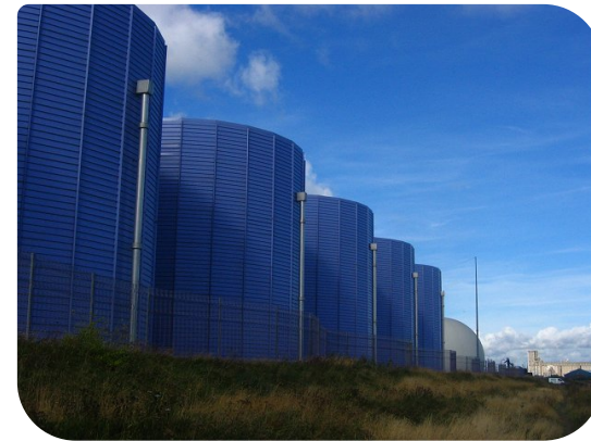
Wastewater Treatment Facility
