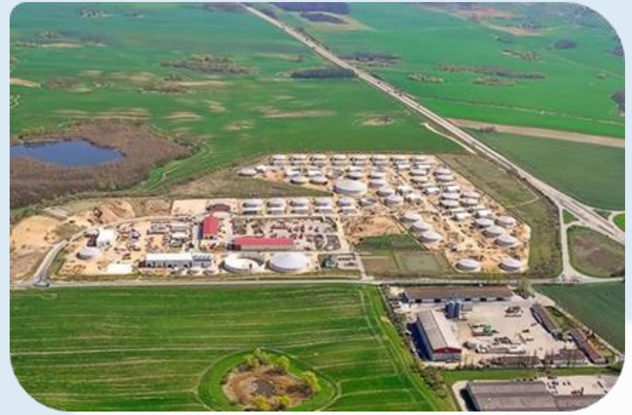
Biogas digester facility powering 50,000 homes
