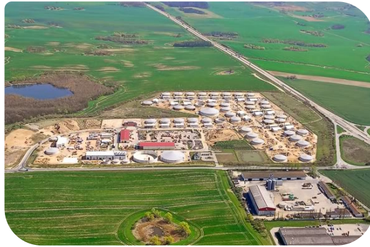
Biogas Digester Facility
