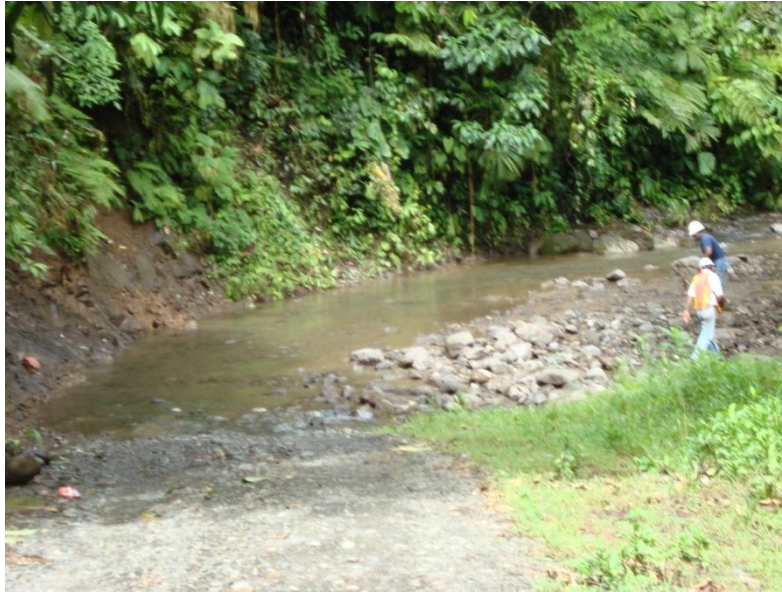
FIGURE 3: ROAD IN EL SILENCIO Road covered in water. (El Silencio, November, 2008)
