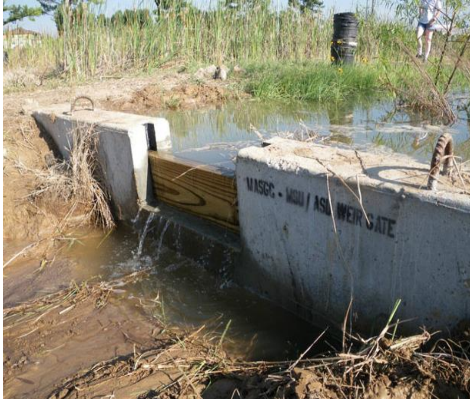
Figure 2.3: A typical flashboard weir (MSU, 2016)
