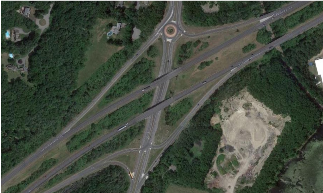
Figure 4: Bird's Eye View of the MA-12 and I-190 Interchange (Google Earth, 2023)
