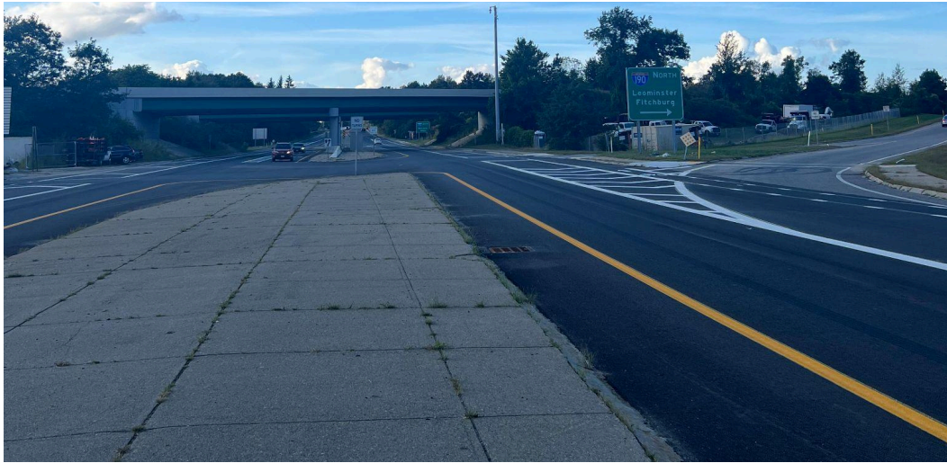
Figure 3: View of Interchange Northbound
