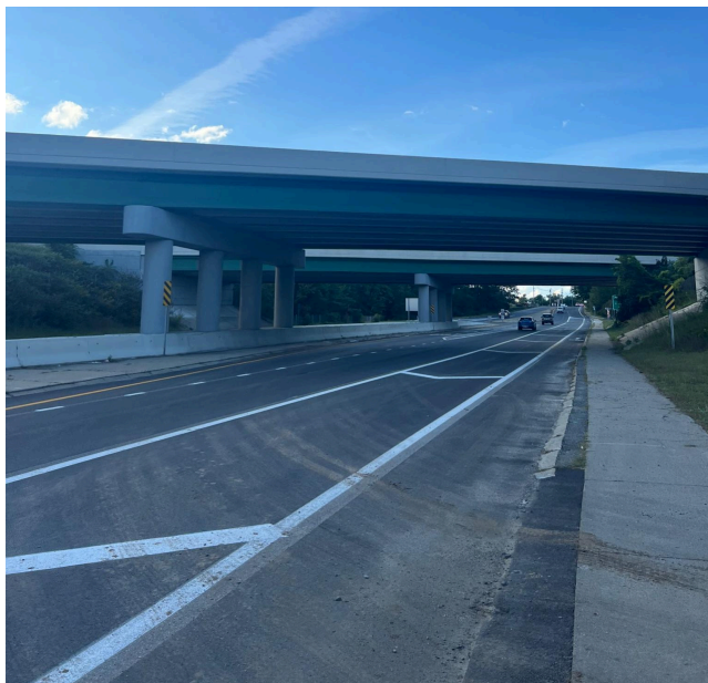
Figure 9: Route 140 North Passing Under I-190 with a Bike Lane on the Right
