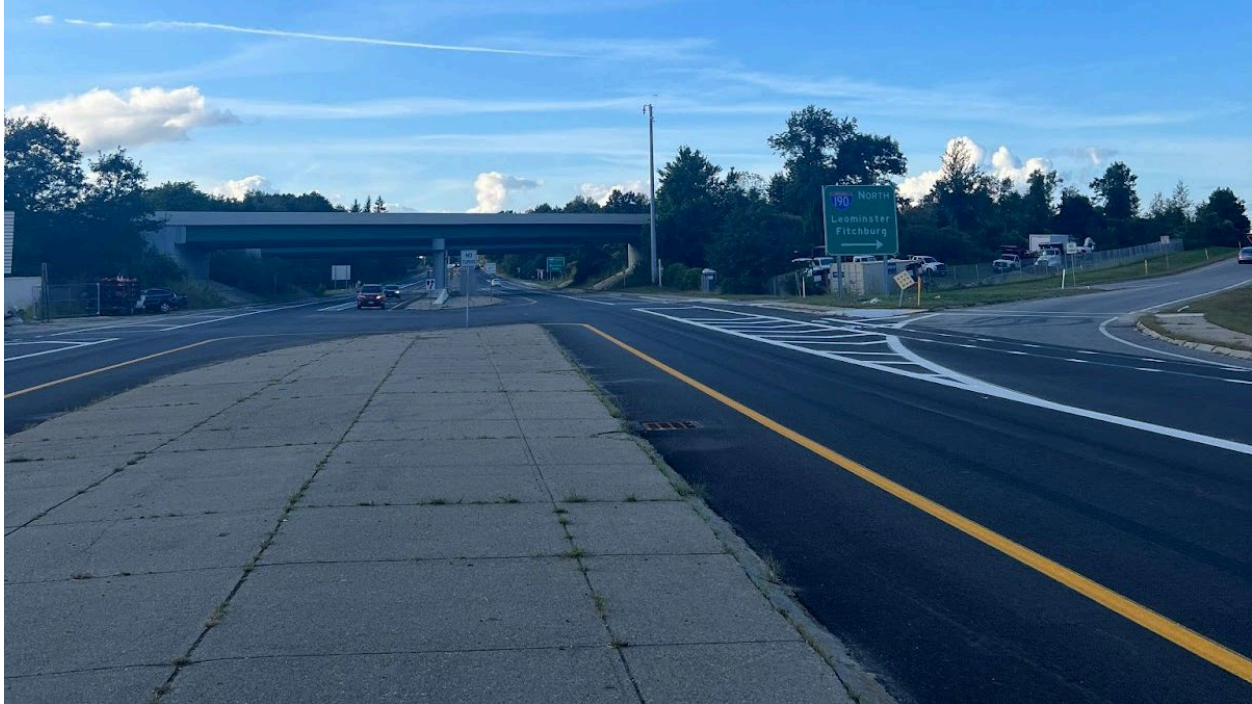
Figure 3: View of Interchange Northbound
