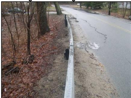
Figure 30 Poor Guardrail
