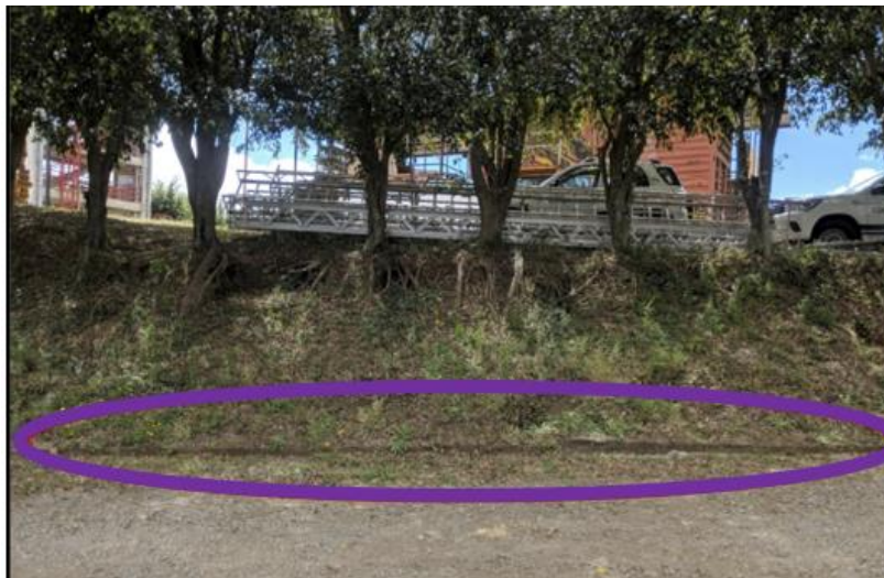
Figure 23: Perspective from behind hill for proposed water storage tank design. Existing water conveyance system is marked in purple.
