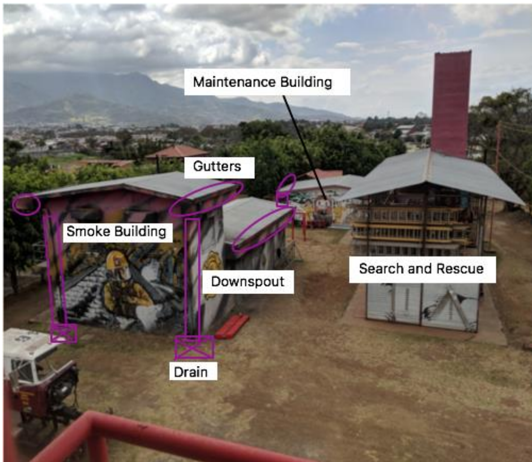
Figure 9: Existing Infrastructure for Smoke Building, Maintenance Building, and Search and Rescue Building
