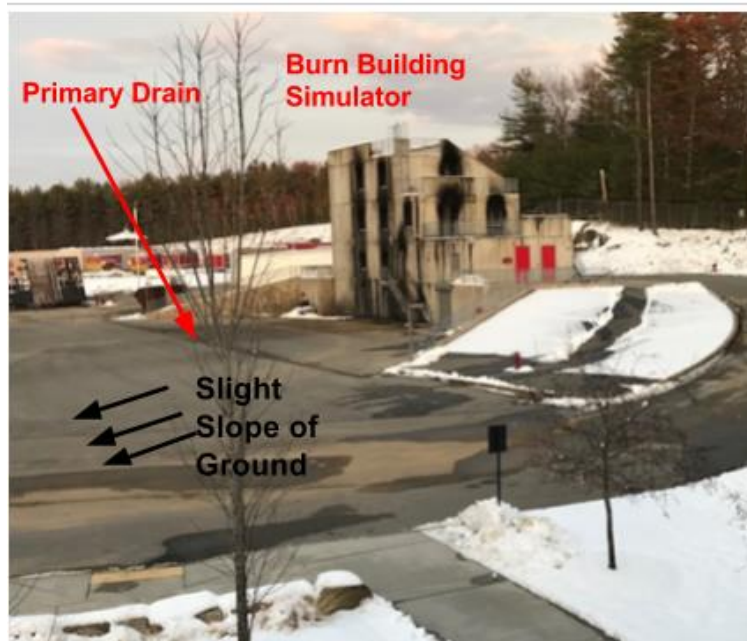
Figure B.3: Image showing the slight slope down from the burn building simulator to the main drains on the campus (image taken by Joe Klucznik)
