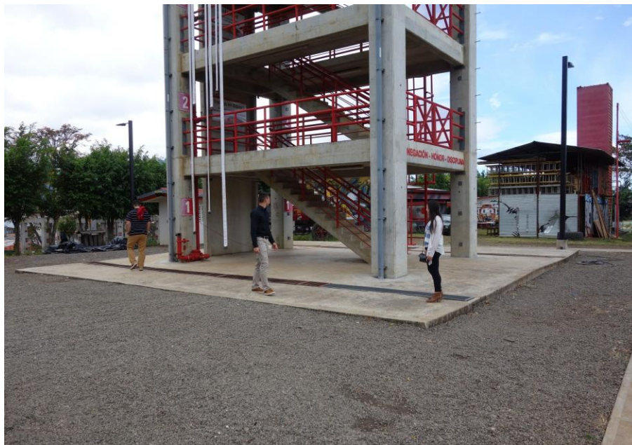
Figure 14: Drain system and gravel around the Training Tower
