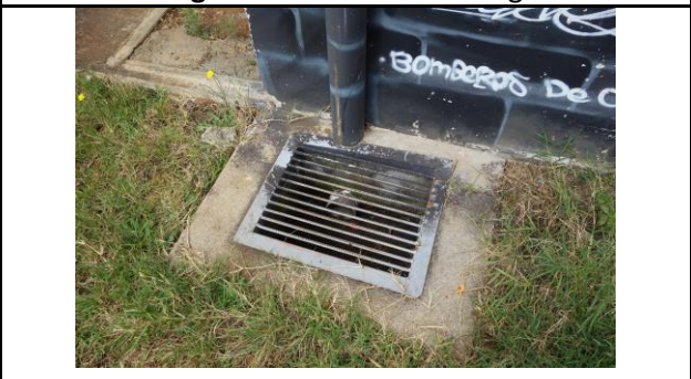
Figure A.4: Drainage system for Smoke Building
