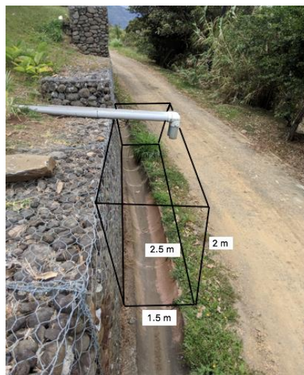
Figure K.2: Proposed location for sediment filter for Administration Area rainwater harvesting tank system
