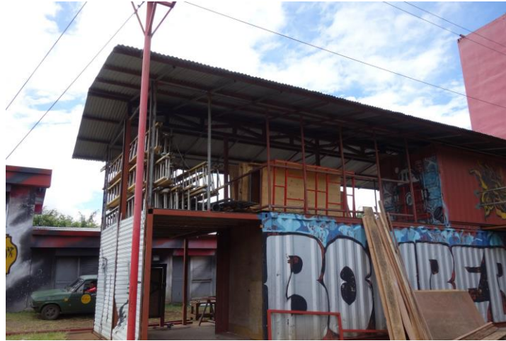
Figure 10: Close-up of Search and Rescue Building
