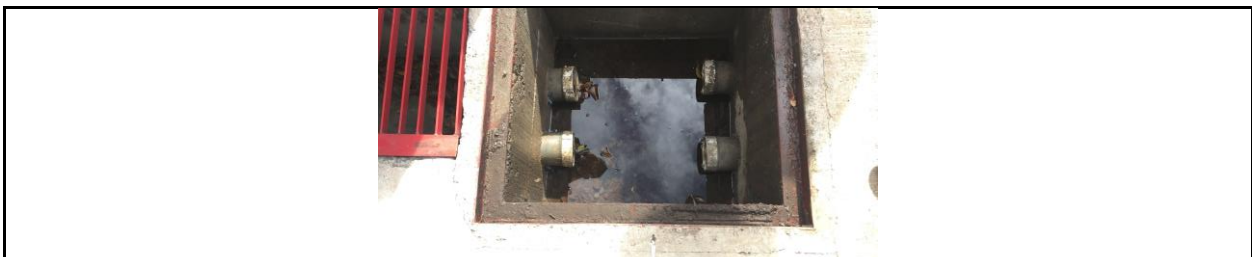
Figure A.11: Original Sediment Traps Underneath Concrete Training Pad
