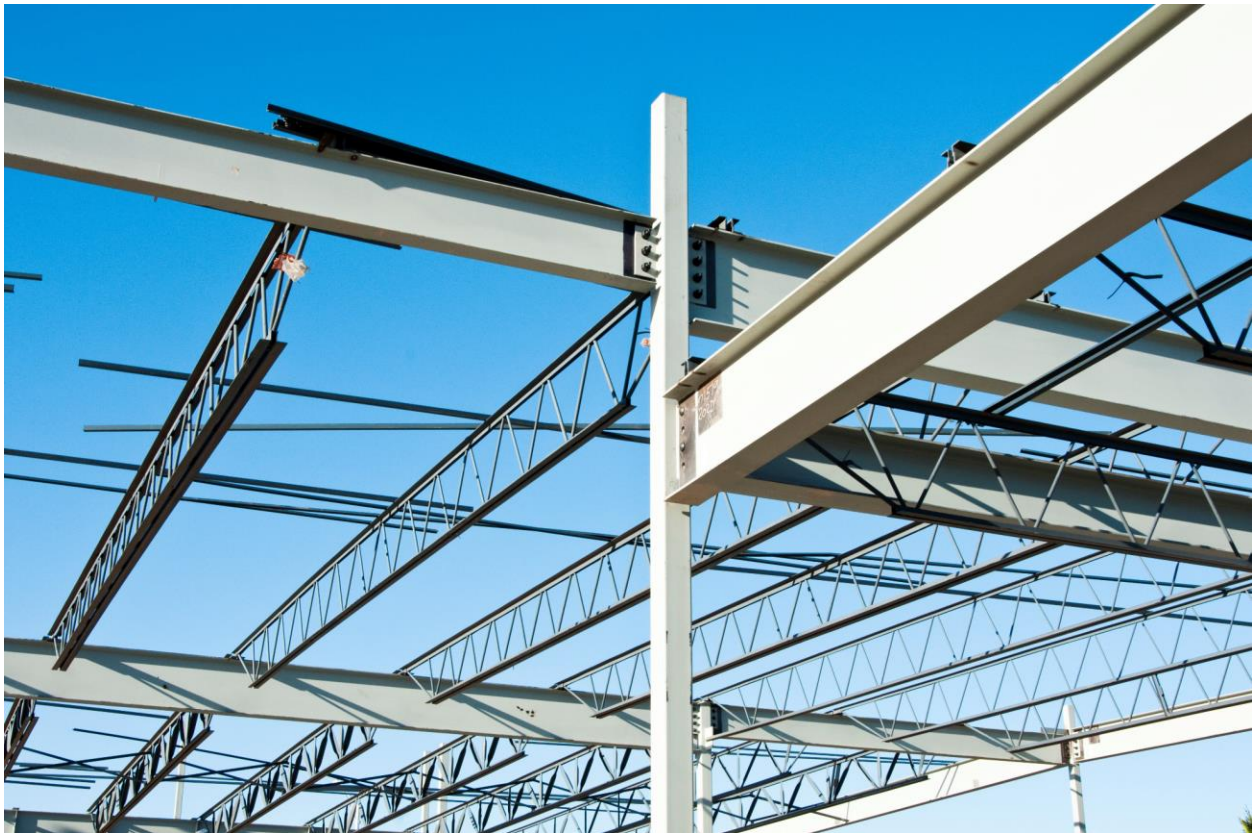
Figure 1: Steel Skeleton of a Building (Metinvest, 2022)
