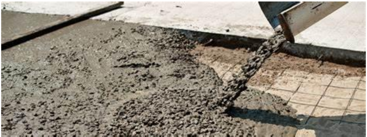
Figure 2: Wet Concrete (Omex, 2021)
