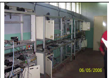
Figure E- 13: Storage of electrical components
