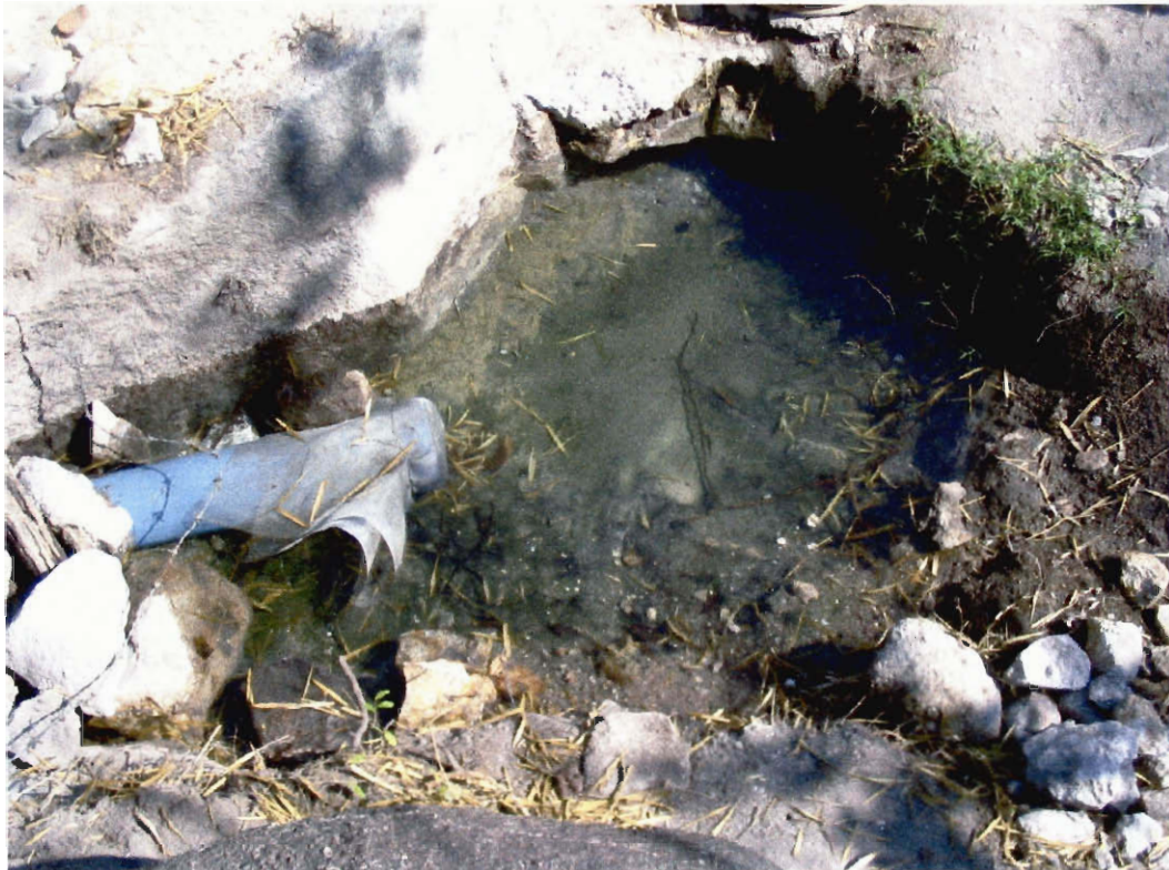
Figure 2.4 - Feeding point for pipe to decorated bathhouse
