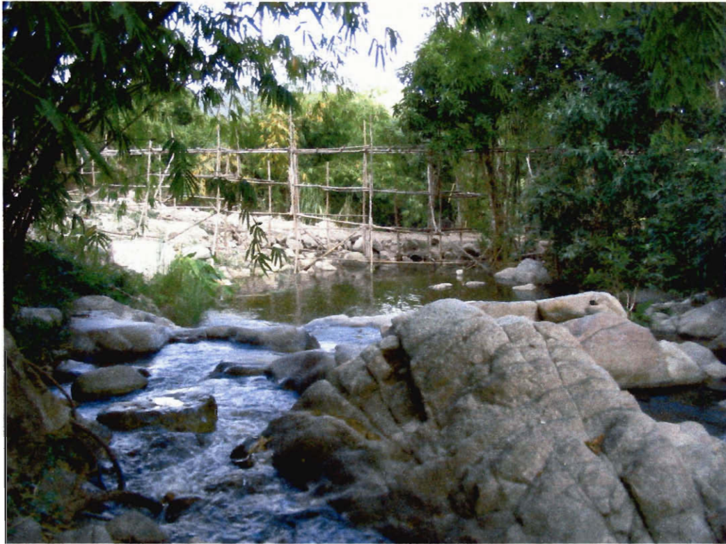
Figure 2.7 - Sling bridge under construction
