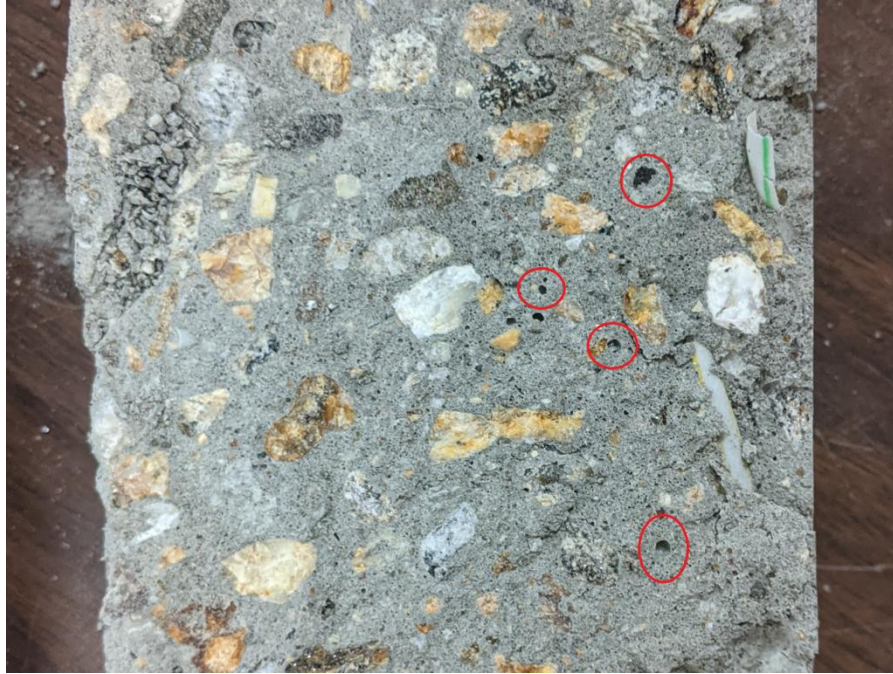
Figure 8: Air pockets within the concrete cylinder.
