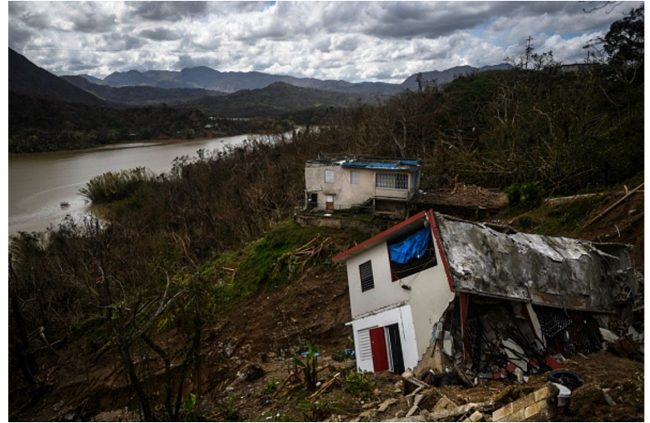
Figure 25. Landslide from Hurricane Maria. (Adapted from Chavez, 2020)
