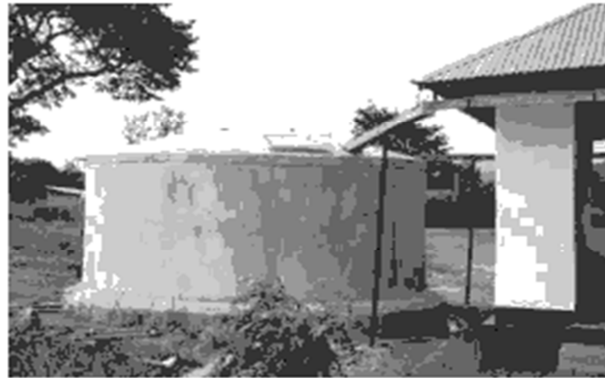
Figure 20 – Ferrocement tank in Ruganzu Village, Tanzania. (Photo credit: DTU) (This is a depiction of a larger water tank. The water vessels that are utilized to store water can range from recycled materials or clay pots, to manmade storage systems)
