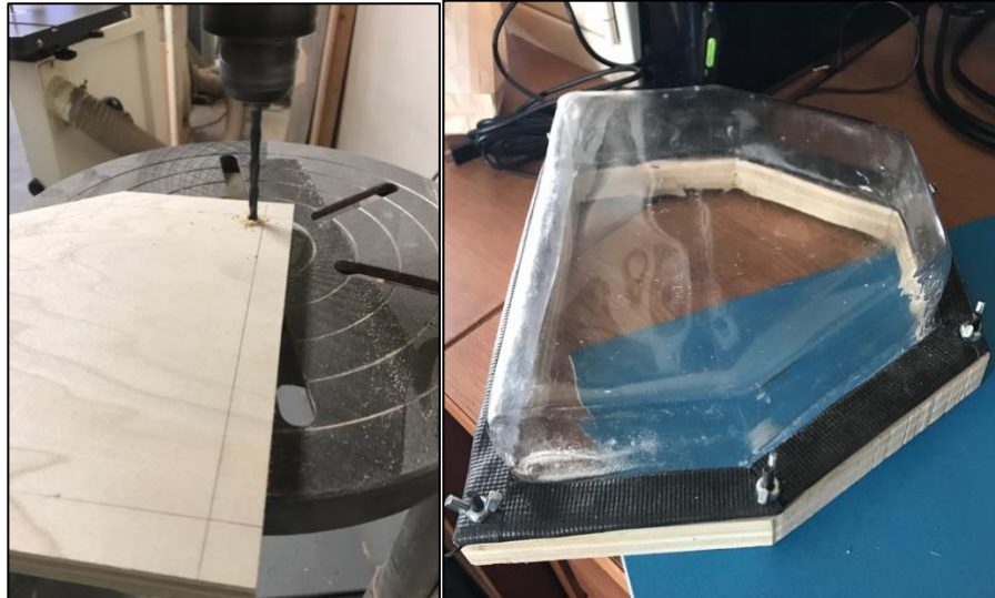
Figure 22: a) Left: Construction of cover base and b) Right: Final assembled cover
