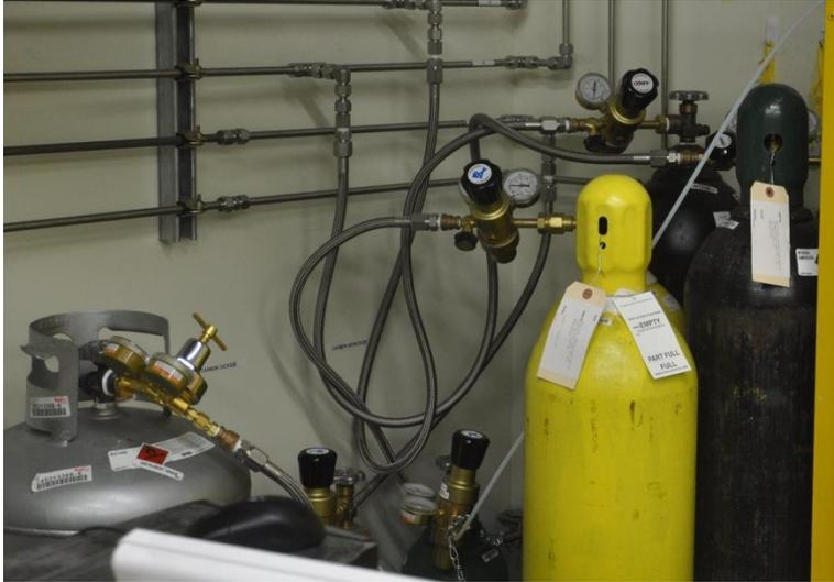
Open valve chain (SS valve, splitting valve)
