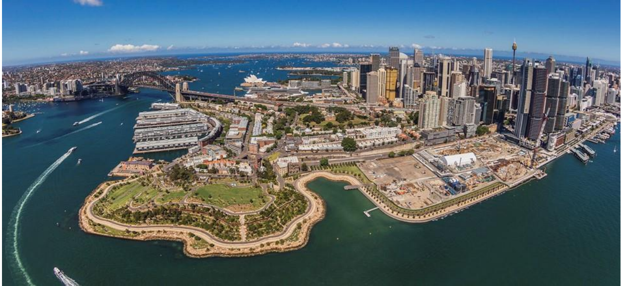
Figure 2.2, Barangaroo development aerial picture (Barangaroo Delivery Authority, 2017c)
