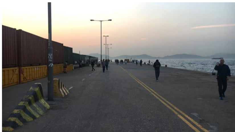
Figure 4.2, Picture of the cargo pier side of Fung Mat Road waterfront
