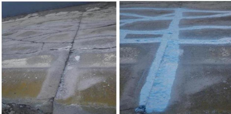
**Figure 3:** Epoxy crack repair. These types of repair are not always long lasting and often have to be reapplied every few years (von Fay, 2015).
