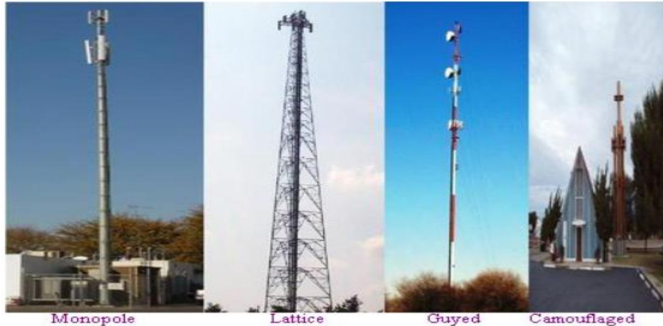
Figure 6: Types of Cell Towers (RF Wireless World- Cell phone tower basics, n.d.)
