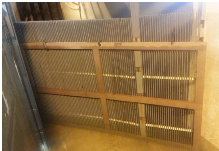
Figure 9 - Debris loading testing completed using wooden planks against the bar rack.
