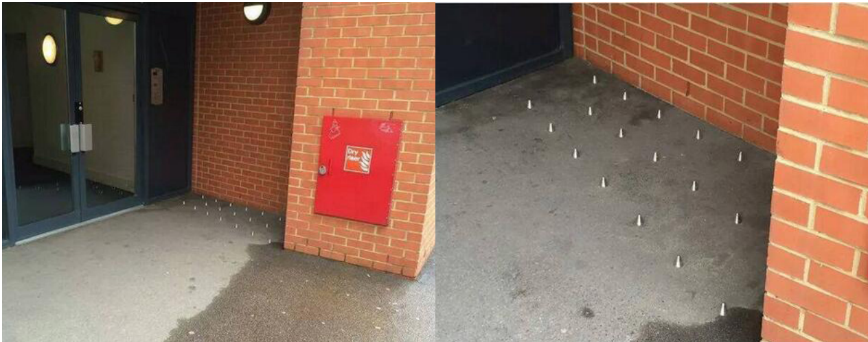
Figures 4 and 5: Spikes installed to discourage homeless use in London, England (ethicalpioneer, 2014).
