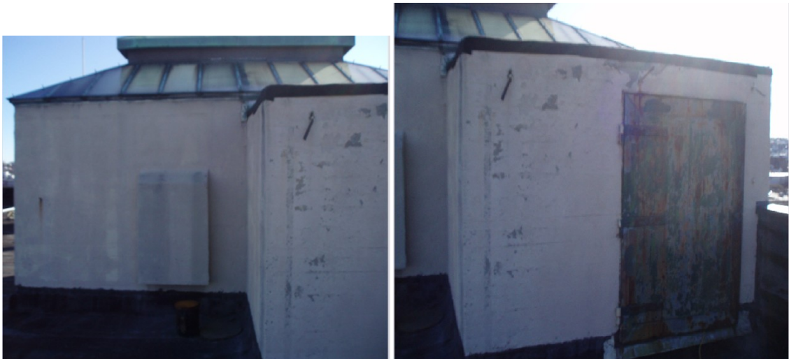
Figures 10b & 10c. Photos of Service Elevator Shaft
