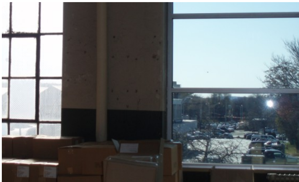
Figure 16b. Photograph of Second Floor New Window and Adjacent Old Window
