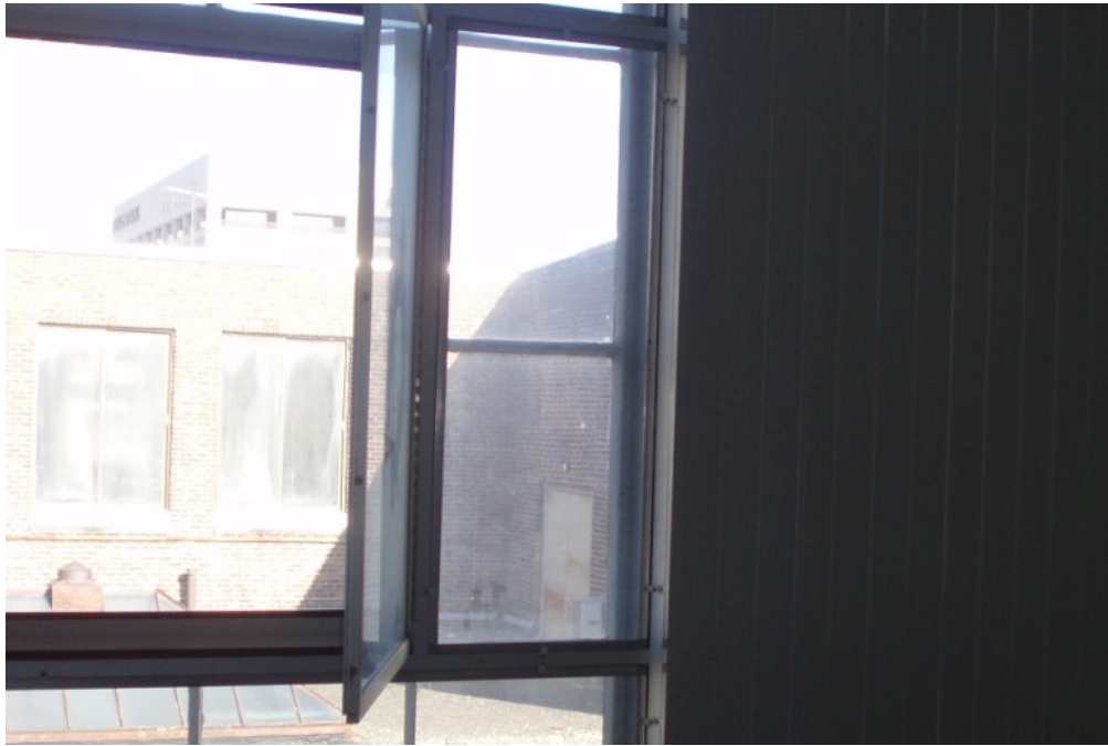
Figure 14b. Photograph of Regular Window, Storm Window, and Blinds
