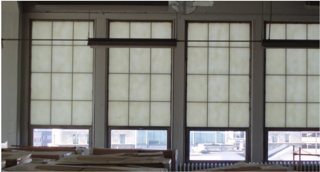
Figure 12b. Photograph of Glazed Window on Seventh Floor
