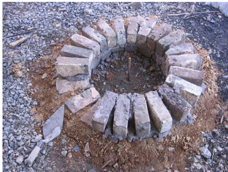
FIGURE 1. THE BASE OF THE FURNACE.
