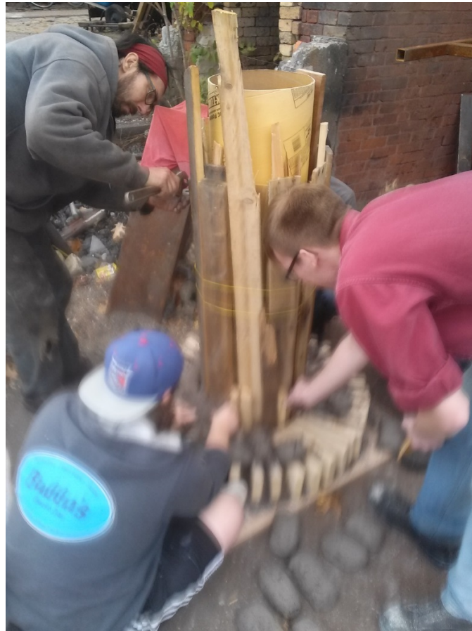
FIGURE 5. LAYERING CLAY ONTO FURNACE SIDES.
