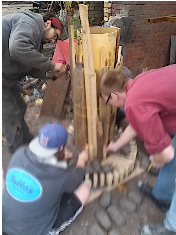
FIGURE 39. LAYERING CLAY ONTO FURNACE SIDES.
