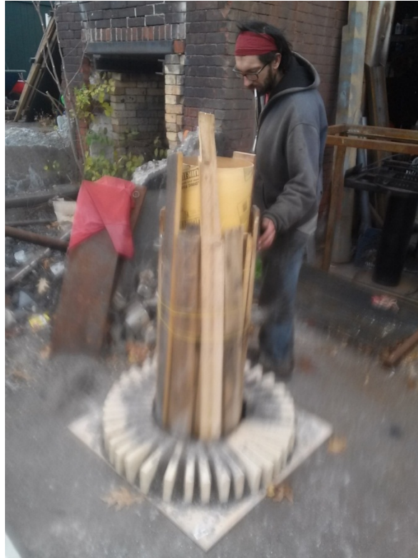
FIGURE 4. FURNACE STRUCTURAL SUPPORT TUBES.
