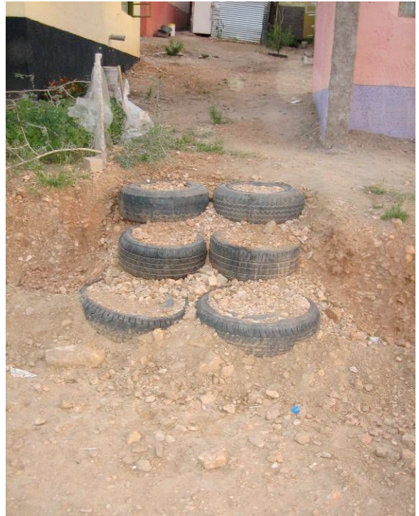
Figure 14: Completed Tyre Steps at Site #4
