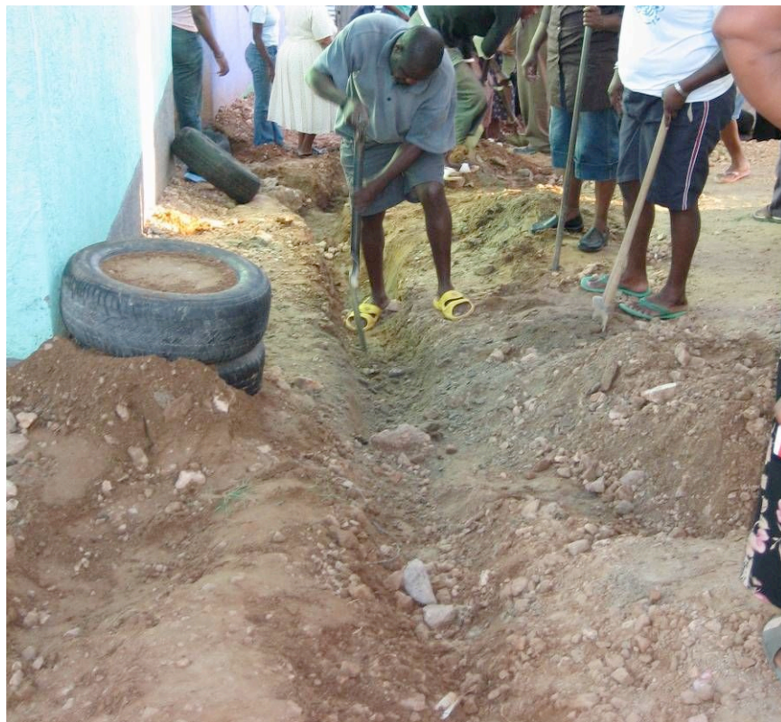
Figure 9: Construction of a Diversion Channel Reinforced by Tyres at Site #2
