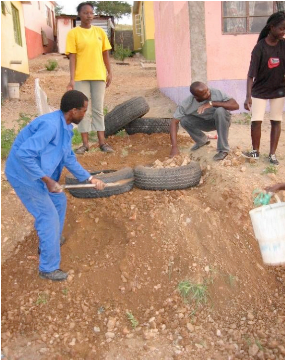
Figure 13: Construction of Tyre Steps at Site #4
