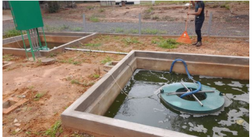
Figure 3: There are two pools that have “good” bacteria, which is responsible for cleaning the water.
