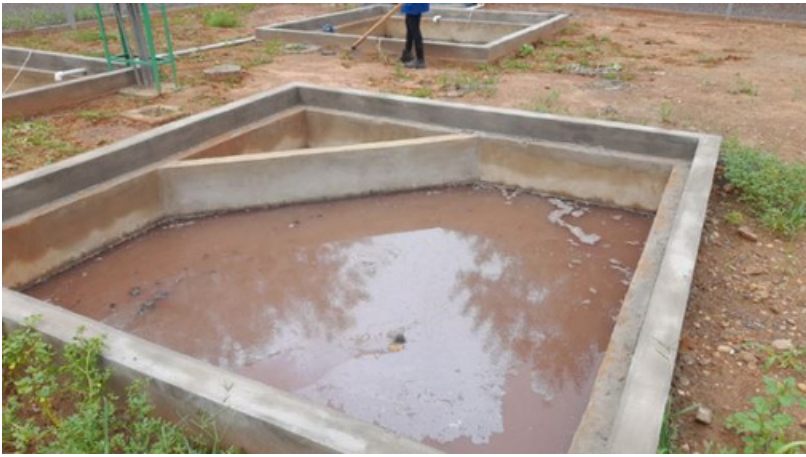
Figure 2: The first pool where the fat is retained from the water.
