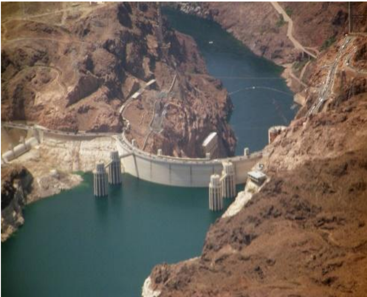
Figure 2.6-1: Aerial Photograph of The of Hoover Dam
