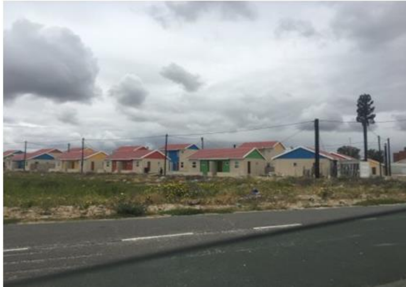
BNG Development in Delft
