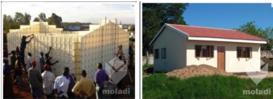
Figure 4: Construction with Moladi Plastic Panels (Moladi, 2018)
