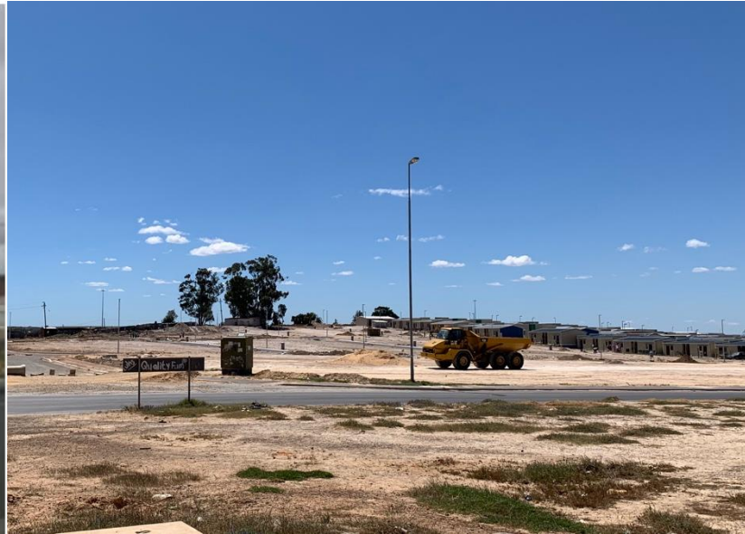
BNG Construction in Atlantis
