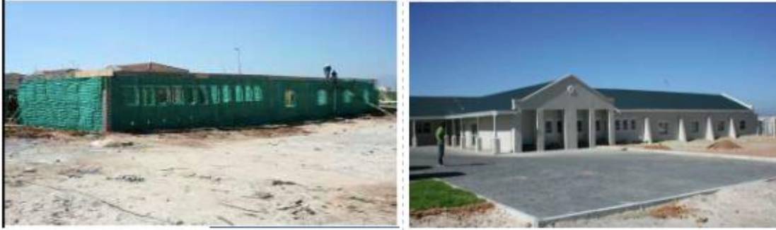
Figure 3: Construction of Sandbag School in Cape Town (EcoBEAM, 2007)
