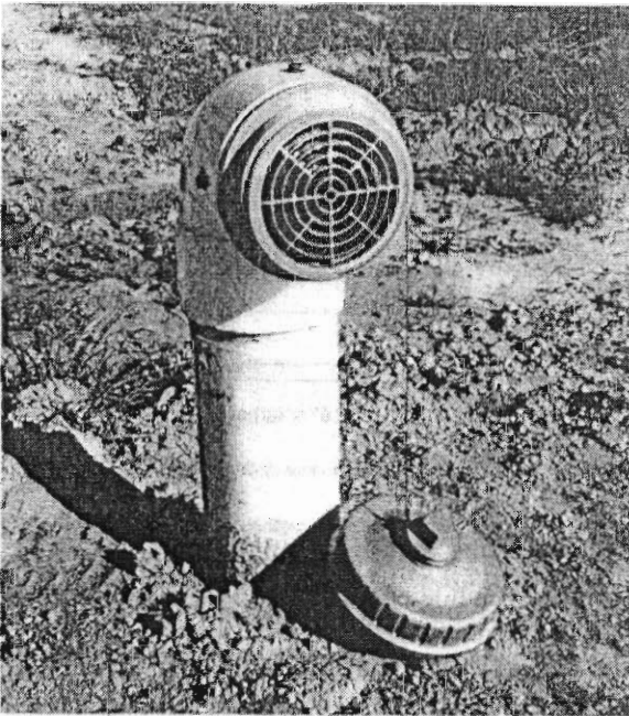
Figure 4-2 – Dry Hydrant
