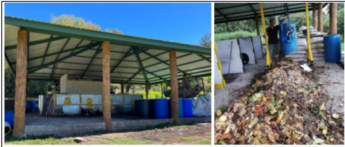
Figure 3.10. Current small-scale productive treatment plant in Monteverde (Welch, 2021).
