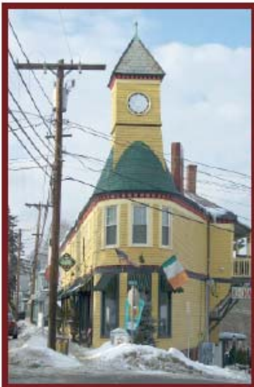
The Flat Iron Building was awarded the Smart Growth award by the Central Massachusetts Regional Planning Commission in 2005.
