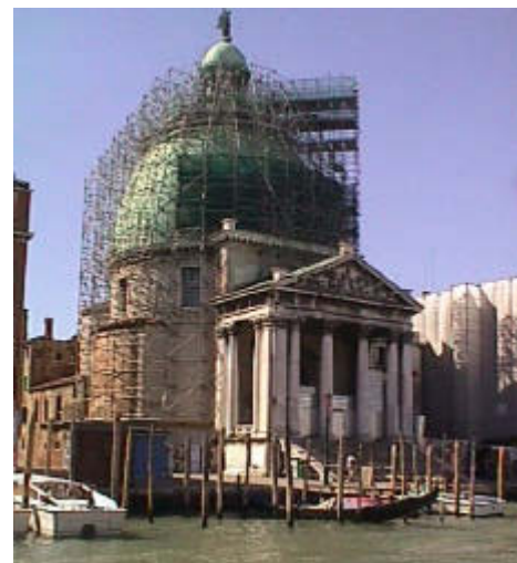
Figure 6: Restoration of Façade of S. Simeone
