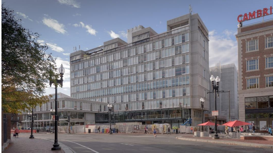
Figure 4: The Smith Campus Center.
