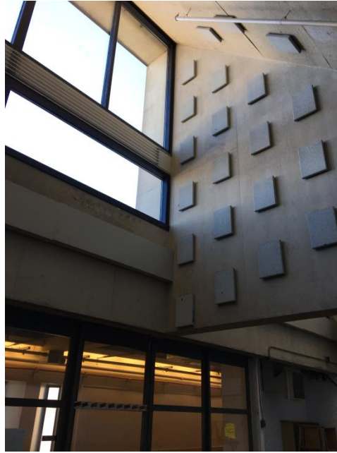
Figure 36: North-facing window and acoustic panels inside one of the studios.
