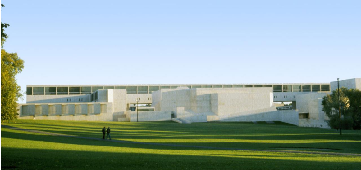
Figure 12: Fine Art Center, North elevation. The windows of the Art Studio are in the back of the center.
