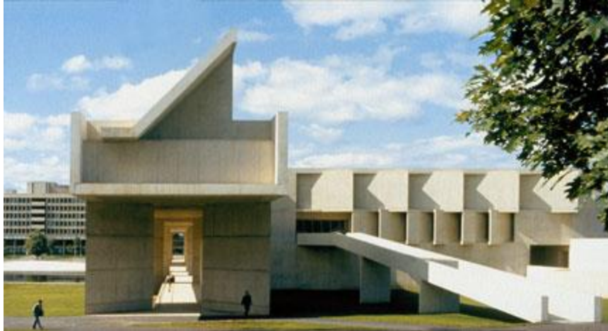
Figure 10: Fine Art Center, East elevation, showing Art Studio Building (left), and Building B (right).
