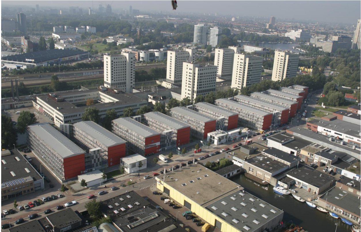
Figure 3.6: The blocks of shipping container units that make up Keetwonen (“A Thousand Strong,” 2014)
