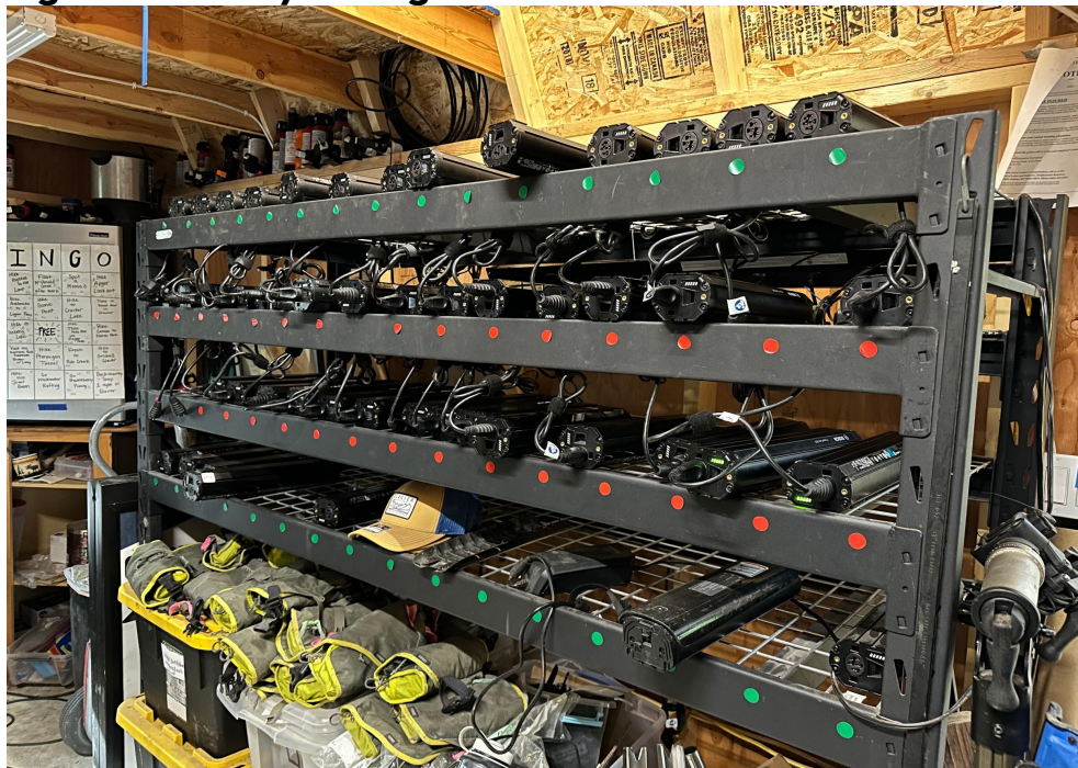
Figure 1. Glacier Outfitters, an activity vendor in Apgar Village that rents e-bikes, has an e-bike battery charging setup showing batteries on a metal rack in a raised storage shed. (J. Wessler, 2023)
