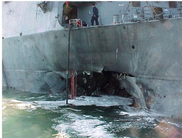
Figure 8. Damage to USS Cole after small craft bombing ([Image of USS Cole], 2012).
