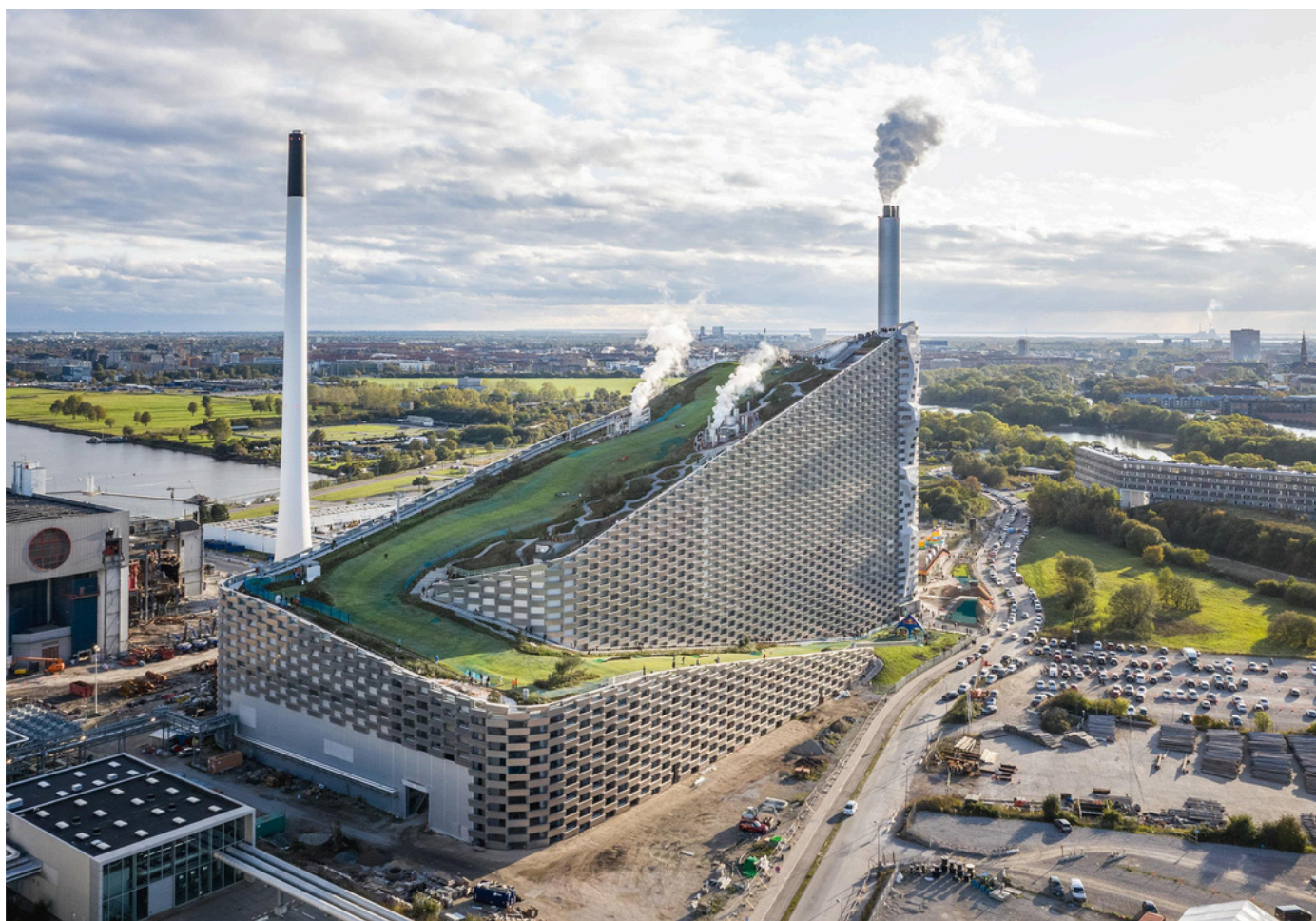
Figure 3. Denmark’s most famous green roof in Copenhagen (Development).
