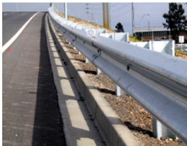
Figure 2-1: Standard W-Beam Guardrail
