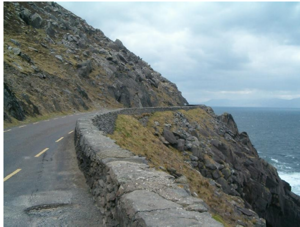
Figure 2-4: Standard Stone Barrier
