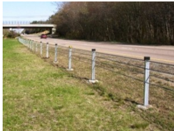
Figure 2-2: Standard Three Strand Cable Guardrail
