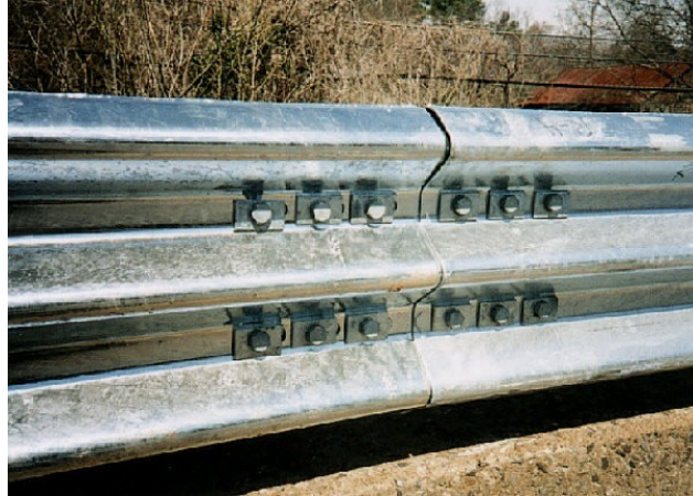
Figure 2-3: Standard Thrie Beam Guardrail
