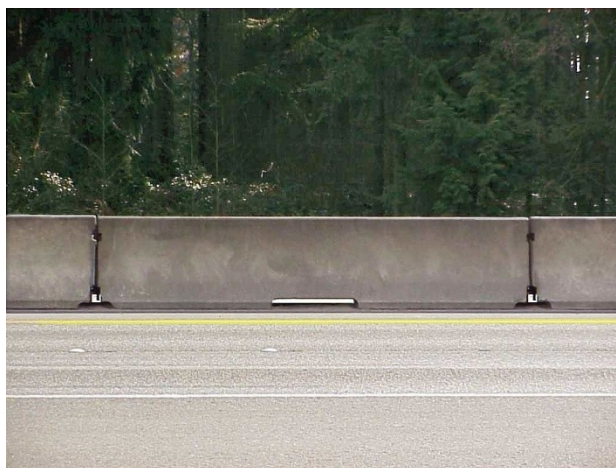
Figure 2-5: Standard Concrete Barrier
