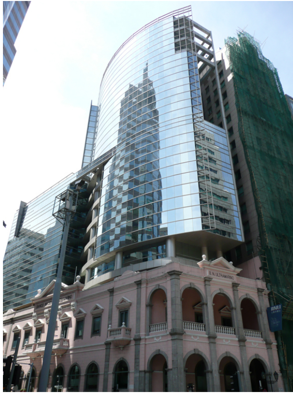
Figure 4: Facade retention on the Banco Nacional Ultramarino, Macao (Hinto, 2007)
