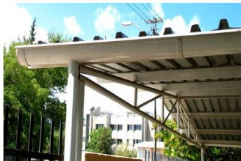
Figure 4.4: Conventional Gutter Conventional gutters are easily accessible from any building supply store in the Windhoek area, at an approximate cost of N$90 for a square, 3.6m long section. Necessary hardware for the installation of a conventional gutter includes a gutter end-piece, which comprises of a down pipe outlet and a water stop,
