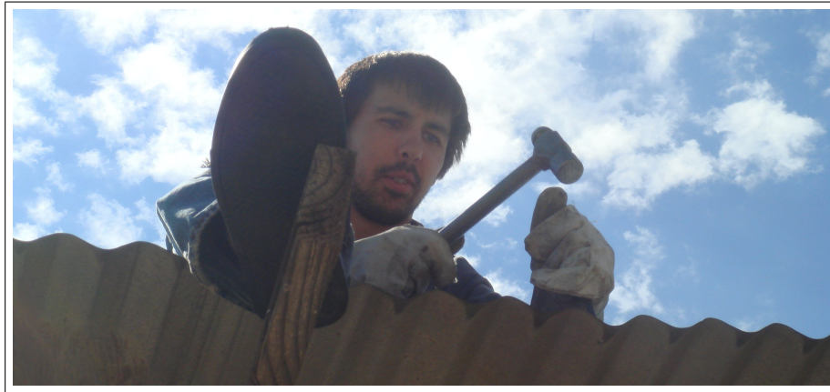
Figure 4.15: Roof Preparation to Hang Guttering
