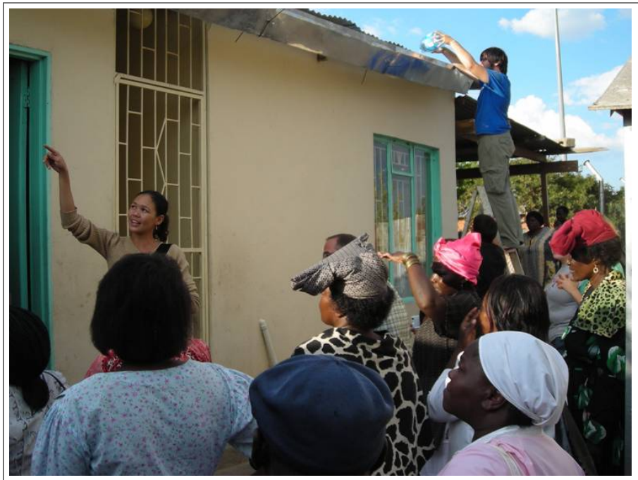
Figure 5.1: Demonstration of Rainwater Harvesting System
