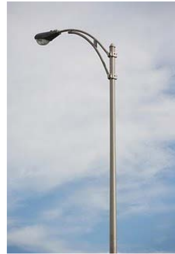
Figure 11: Example of a Type V pole
