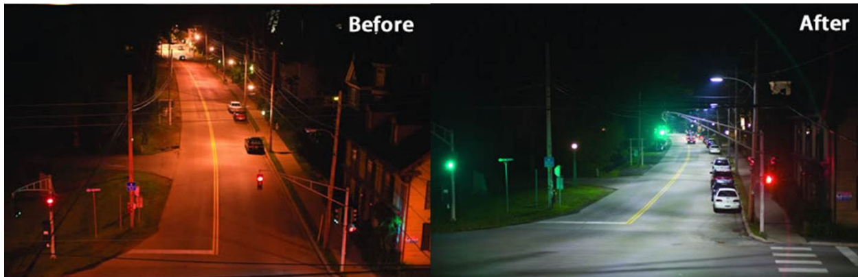
Figure 5: Annapolis Royal, Nova Scotia, before and after the installation of LED Roadway Lighting LED fixtures.
