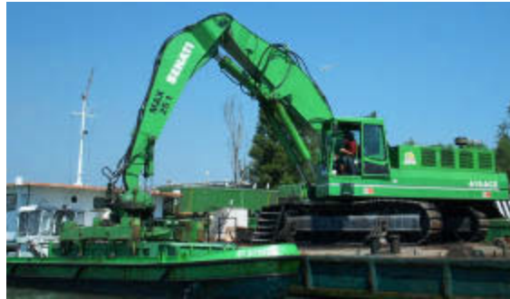
Figure 4.10: Crane lifting insert from garbage boat
