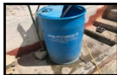
Figure 12: Corroding pipe (top) and chemical container being used for water storage
