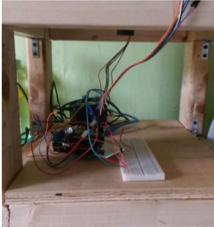
Figure 44: Console Fixture Electronics Housing Box
