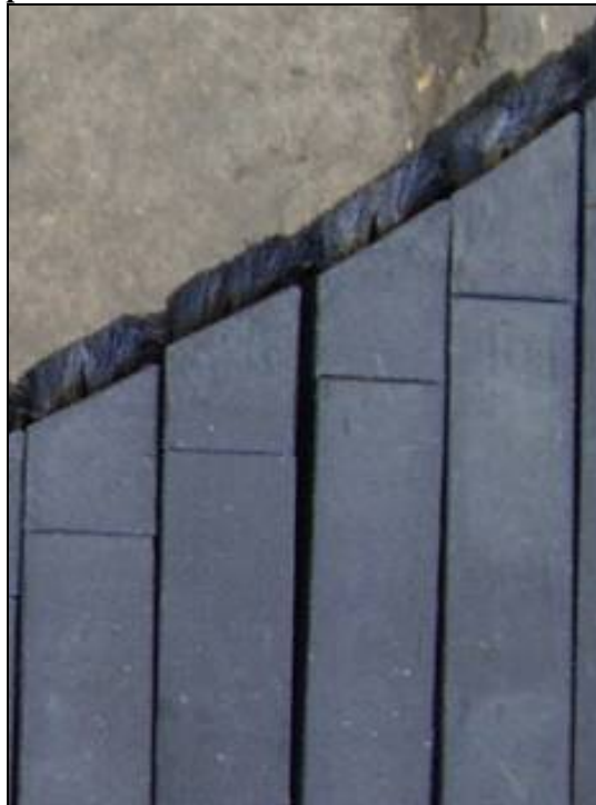
Figure 8: Segment Close-up (top view). Note bristles on end of each segment.
