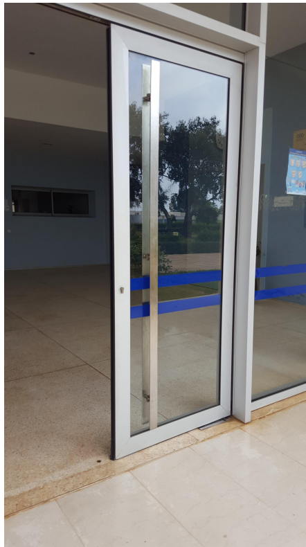
Figure 4.7. A door in the entrance of the Pôle Formation Professionnelle.
