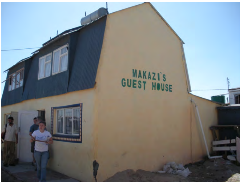
Makazi's Guest House of the Indlovu Project, Monwabisi Park
