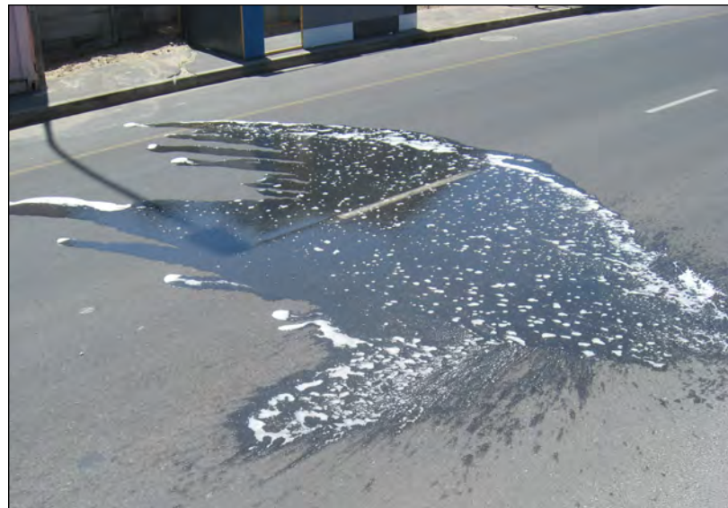
Improper disposal of wastewater often causes extensive erosion problems
