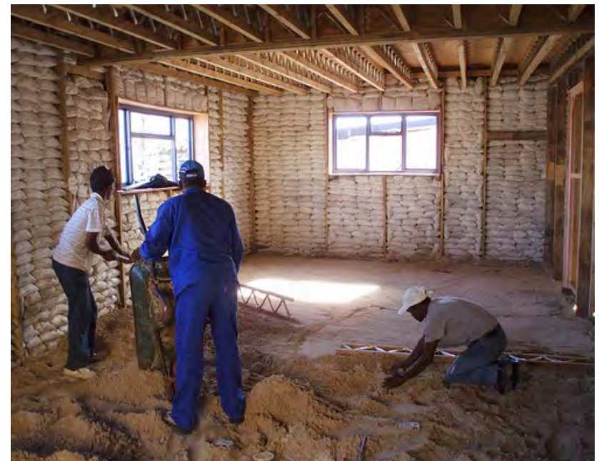
The backpacker's Lodge being constructed of EcoBeams and sand bags
