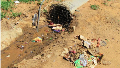
Figure 8: Trash cleaned out of sewage pipe in J-Section as routine maintenance
