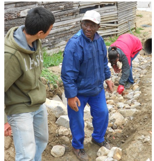
Figure 3: Working on the J-section channel
